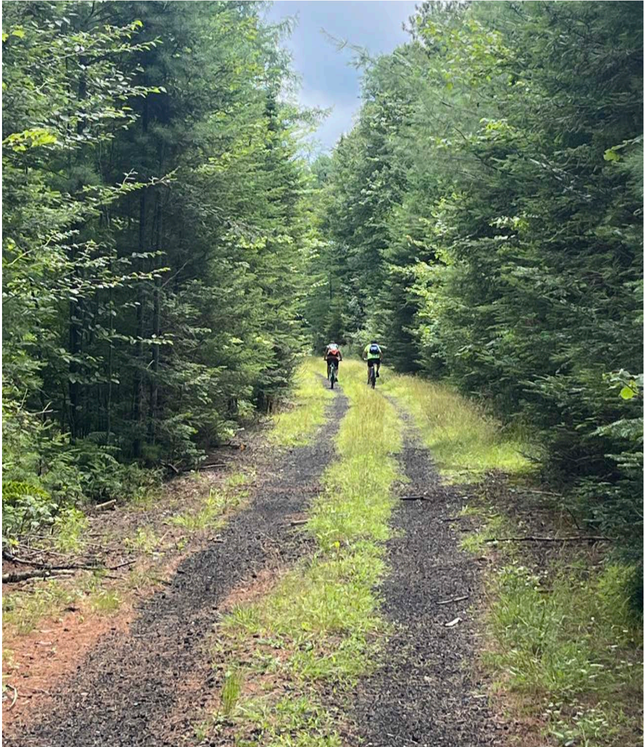
This photograph was taken on Phase 3 of the Adirondack Rail Trail to the west of Rollins Pond. It shows that the existing railbed is approximately 10 feet wide or more, there is cleared space on both sides of the railbed, and there is plenty of width for two bicyclists to travel side by side.
