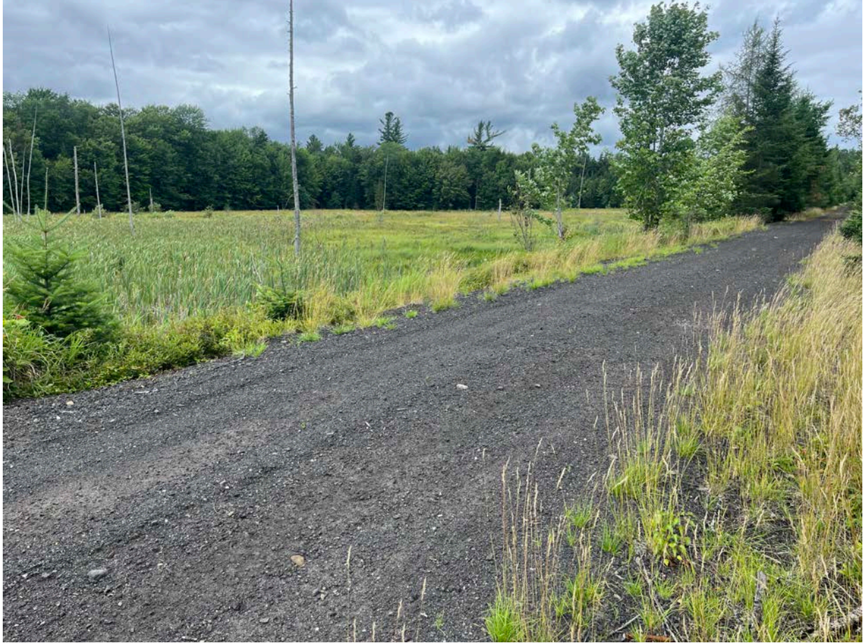
This photograph was taken on Phase 3 of the Adirondack Rail Trail to the west of Rollins Pond. It shows that the existing railbed already has a stone surface that is approximately 10 feet wide or more, and that there is cleared space on both sides of the trail.
