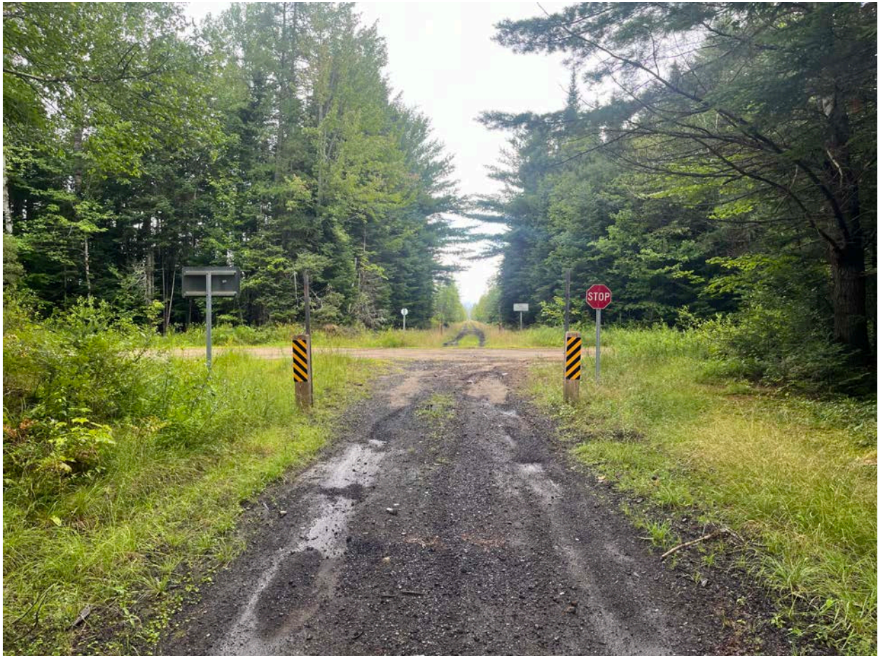
This photograph was taken on Phase 3 of the Adirondack Rail Trail at the intersection with Lead Pond Road. It shows that the existing railbed is approximately 10 feet wide or more and there is plenty of cleared space on both sides of the railbed. The bollards and signage are already in place.
