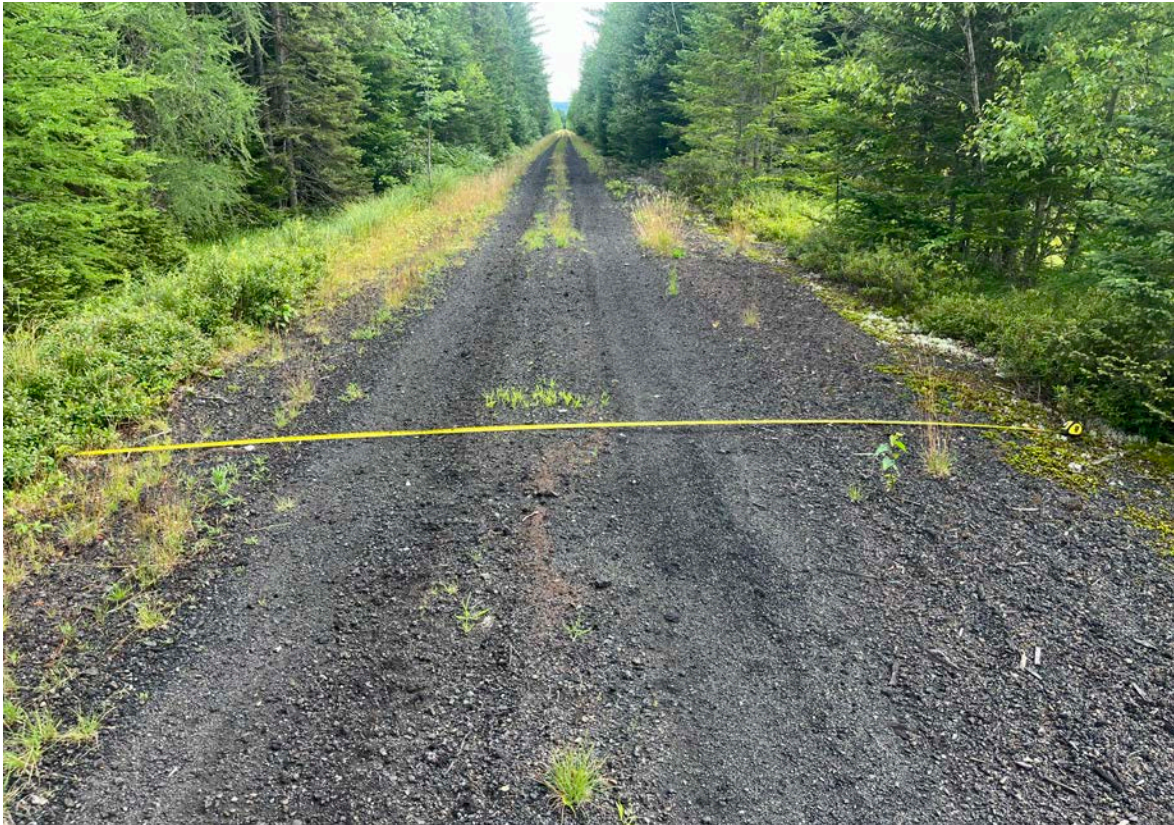
These two photographs were taken on Phase 3 of the Adirondack Rail Trail and are representative of the entire length of trail, which has an existing railbed that is approximately 10 feet wide.
