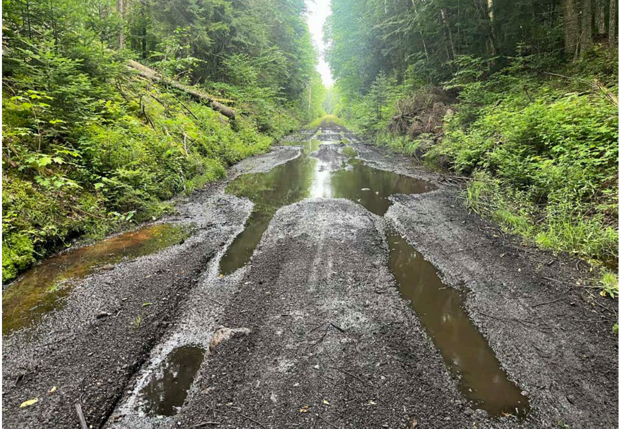
This photograph was taken on Phase 3 of the Adirondack Rail Trail to the west of Rollins Pond. It shows that the existing railbed is approximately 10 feet wide or more and that it is wide enough for motor vehicles to travel down the middle with clearance on both sides.
