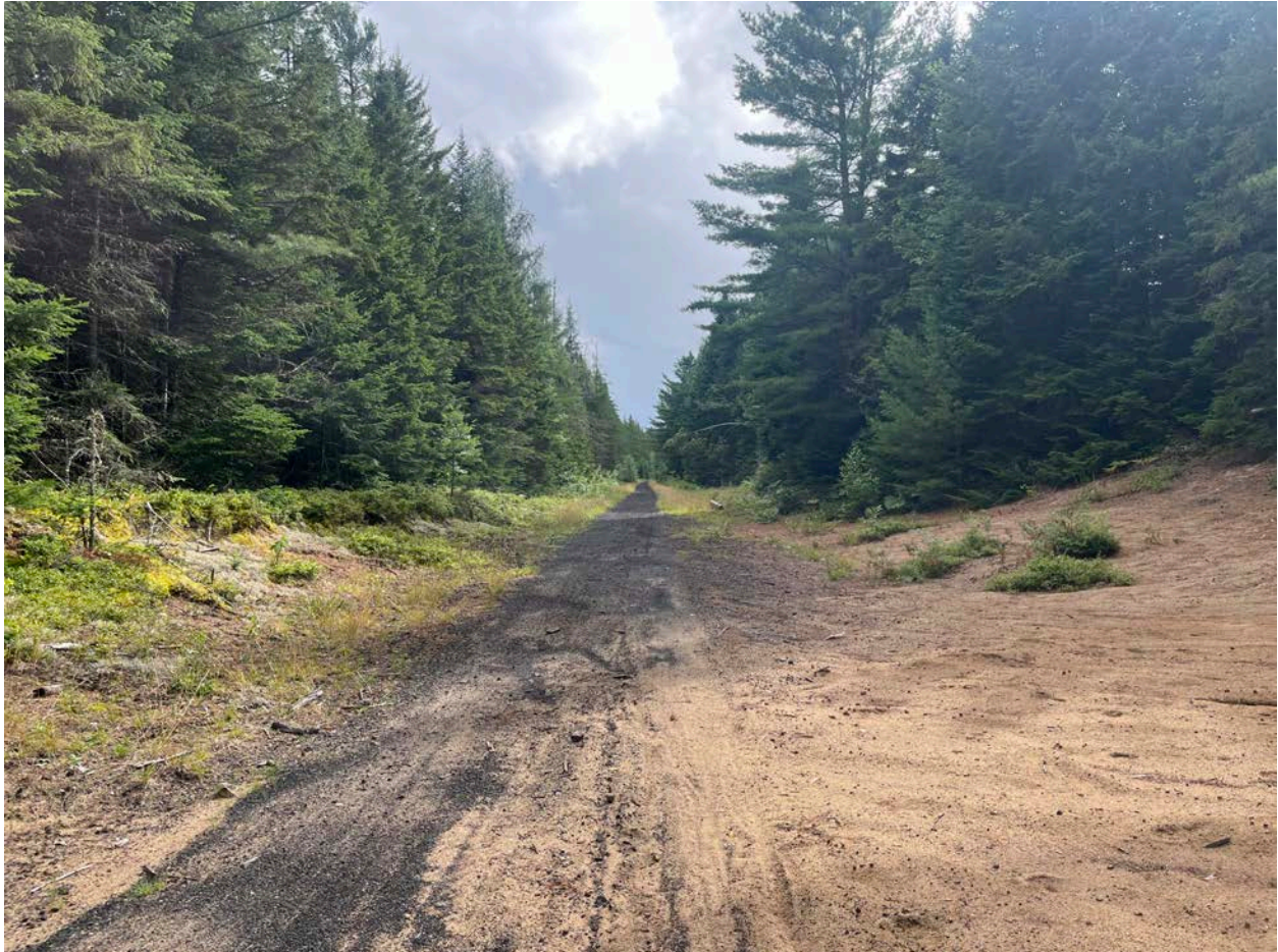
This photograph was taken on Phase 3 of the Adirondack Rail Trail where the trail comes close to, but does not intersect with, Lead Pond Road. It shows that the existing railbed is approximately 10 feet wide and there is plenty of cleared space on both sides of the railbed.
